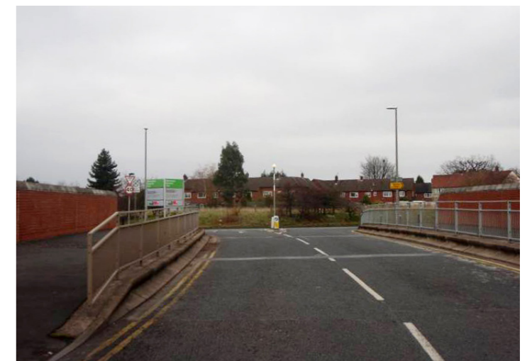
24. Ringway Road Bridge Looking North
