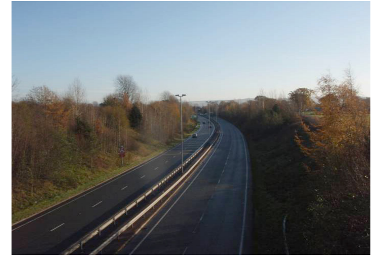
16. Moorfield Bridleway No. 3 (Structure No. 836) Looking East
