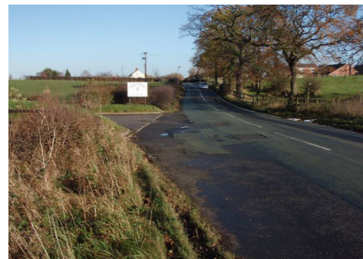
11. Woodford Road to Southwest of Proposed Bridge Looking Northeast
