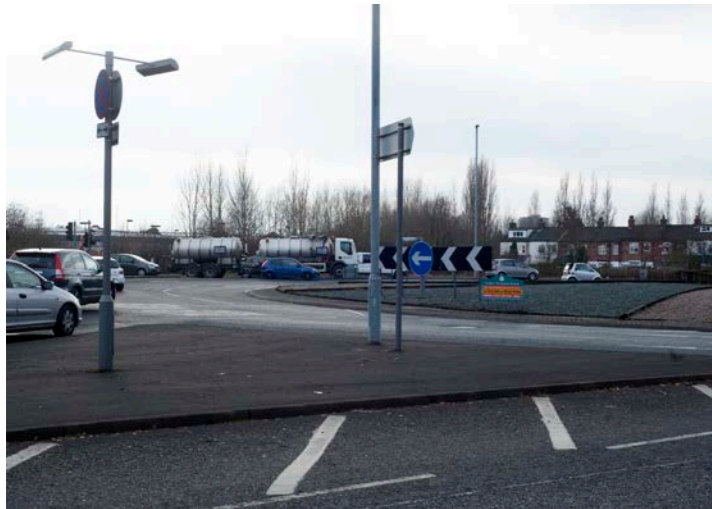
17. Stanley Road Roundabout Looking South
