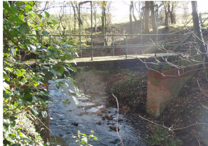
5. Norbury Brook Looking West at Fernlea Footbridge (Structure No. 597)
