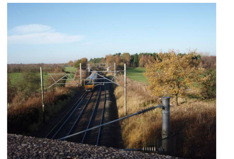
12. Woodford Road Bridge over WCML Looking Northwest
