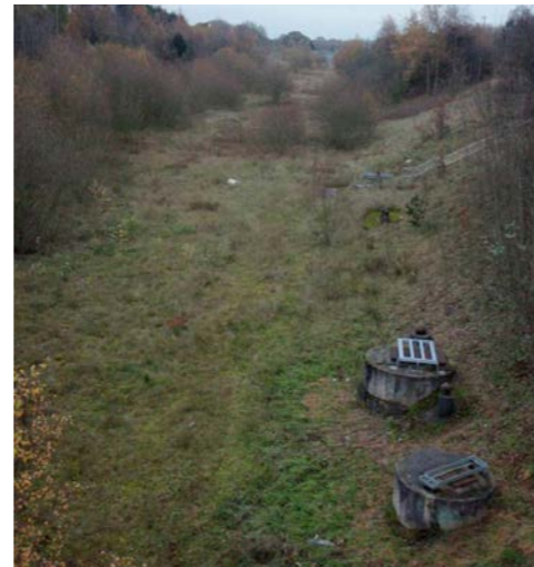
18. Wilmslow Road Bridge (Structure No. CB2320) Looking East along the A555
