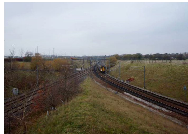
23. Styal Road Looking West along the Airport Spur
