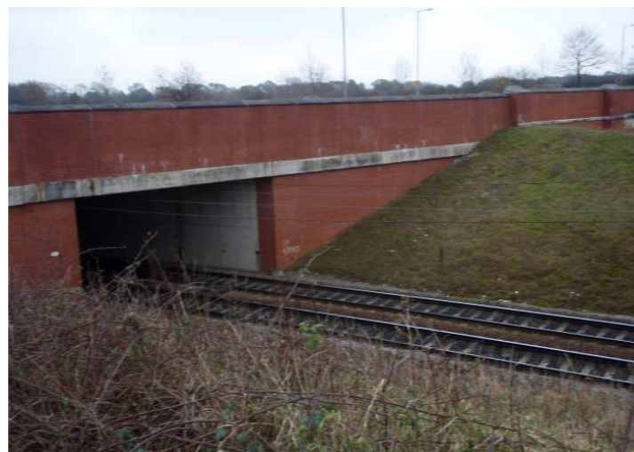
22. View Looking Southeast on the Northern Styal Road Overbridge (Structure No. 526)
