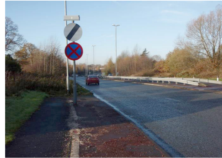
15. Woodford Road, Bramhall Looking West Along A555
