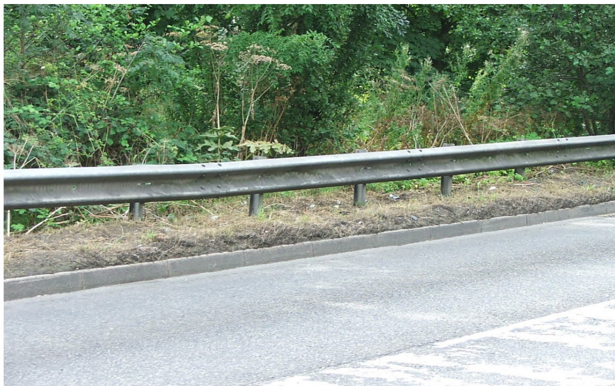
TENSIONED CORRUGATED BEAM
