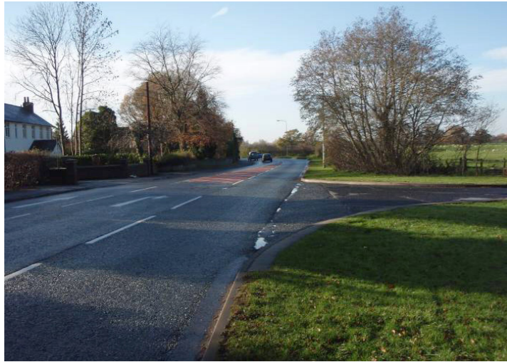
13. Chester Road at Proposed Junction Looking West
